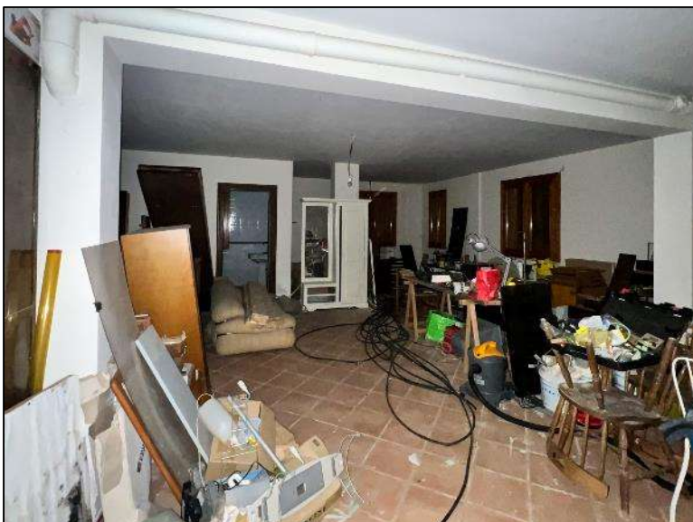
Int. 1 – Piano seminterrato – Locale cantina
